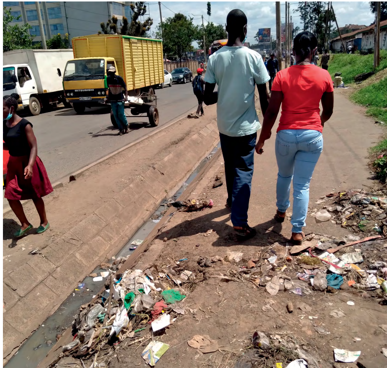
Open drainage and garbage strewn on footpath, Landhies Road. © CDKN.
