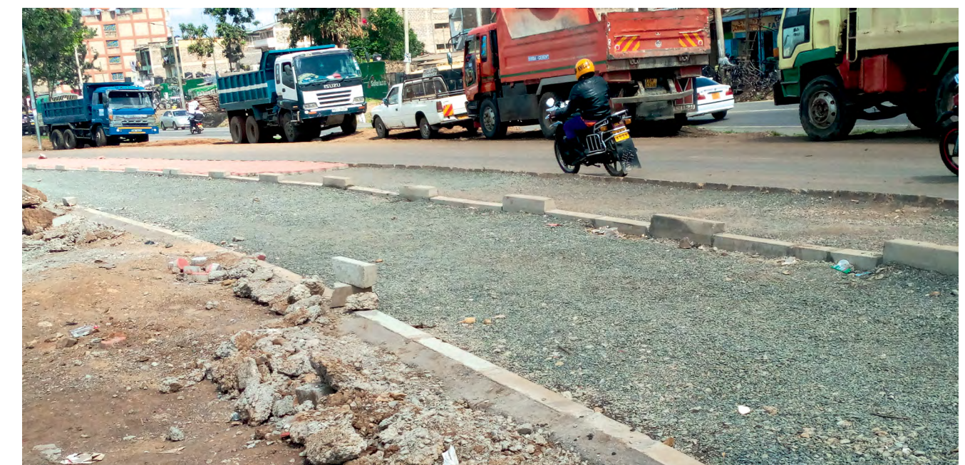
Ongoing road works on footpath, Kangundo Road. © CDKN.
